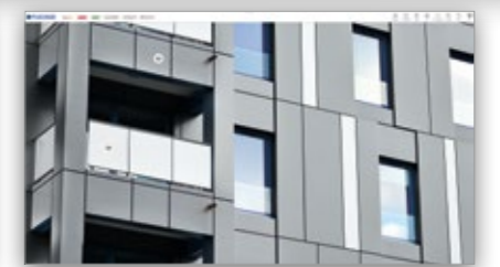
Balconies and parapets
