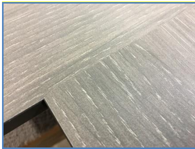
Figure 8/9: Corner connection – top of panel
